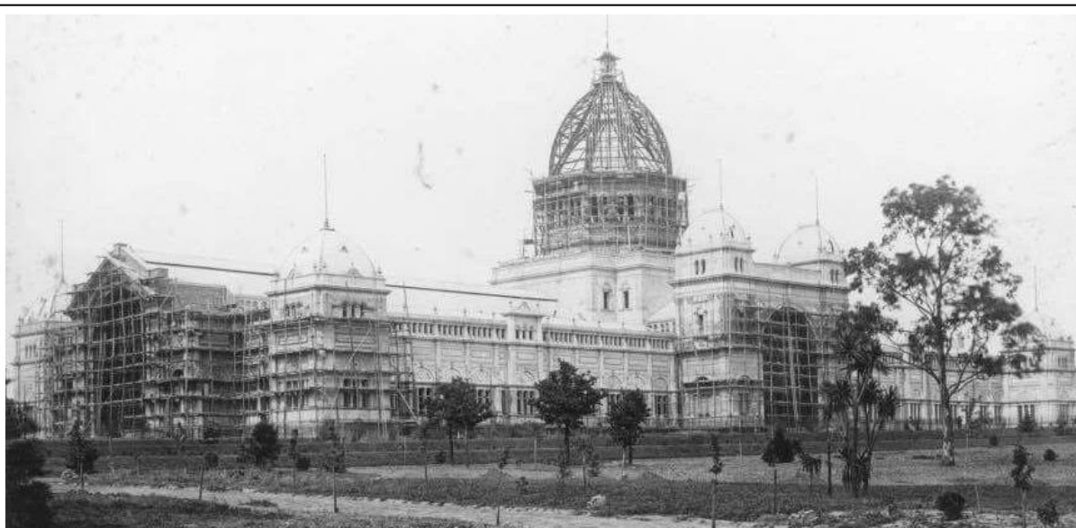
The Exhibition Building under construction in 1879. (Photo: State Library of Victoria)
