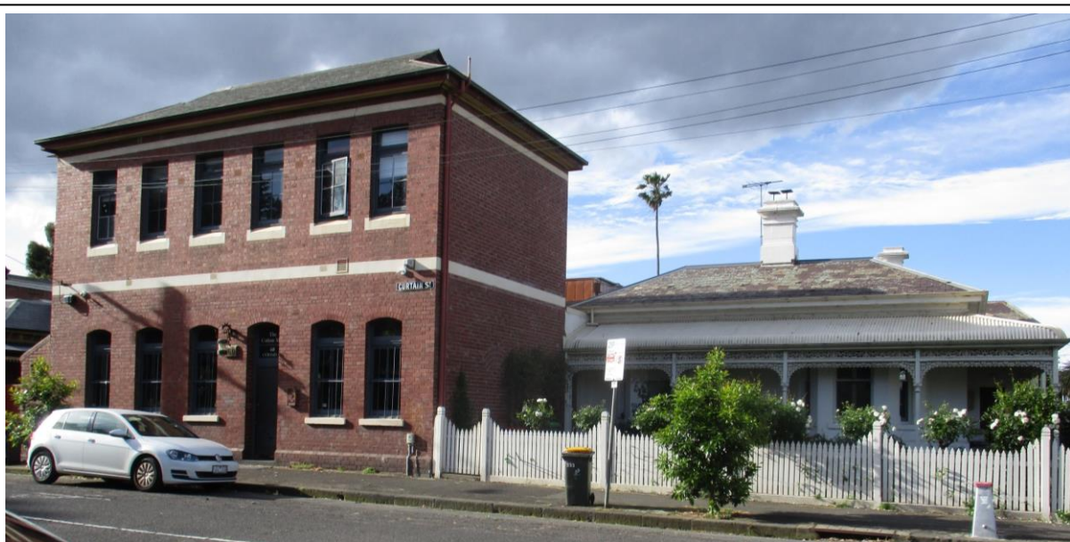
The Cotton Mill, 60 Curtain Street, North Carlton and adjoining house. (Photo: CCHG).
