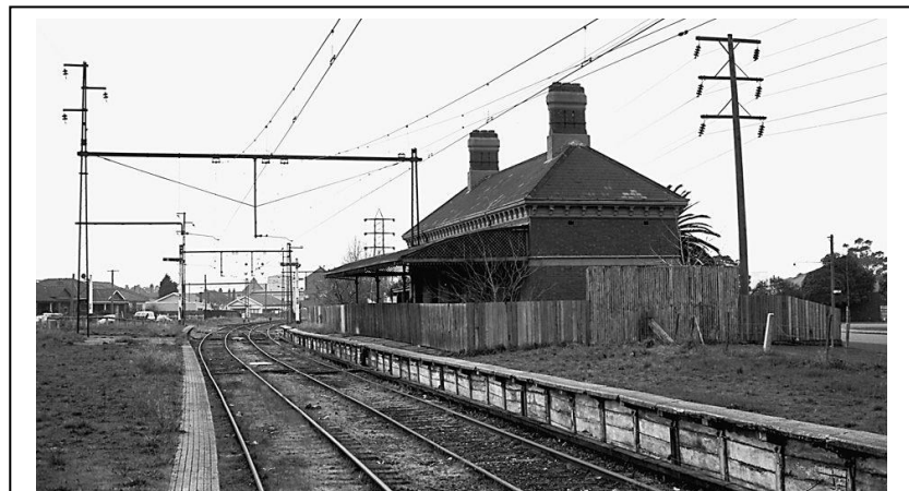
The North Carlton railway station in 1963. The rails, wires and platform were still in place, but the building had been converted to a home for a railway worker and his family. (Photo: John Thompson)
