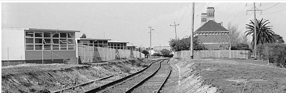
For several years while the Princes Hill High School was being re-built in Arnold Street, Forms 3 and 4 were located in these portable classrooms on disused railway land in Park Street, Princes Hill. (Photo courtesy John Thompson)
