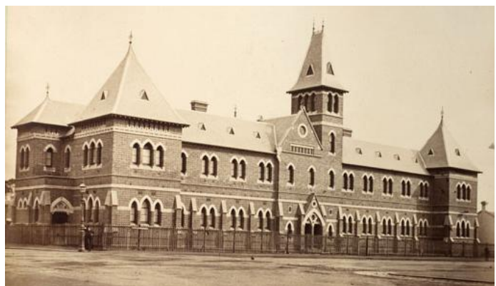
The Faraday Street State School, which is still serving the Carlton community as the Kathleen Syme Library and Community Centre. (Photo: State Library of Victoria)
